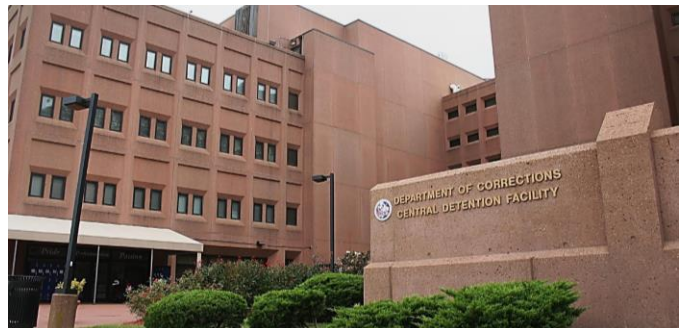
Central Detention Facility (CDF)
